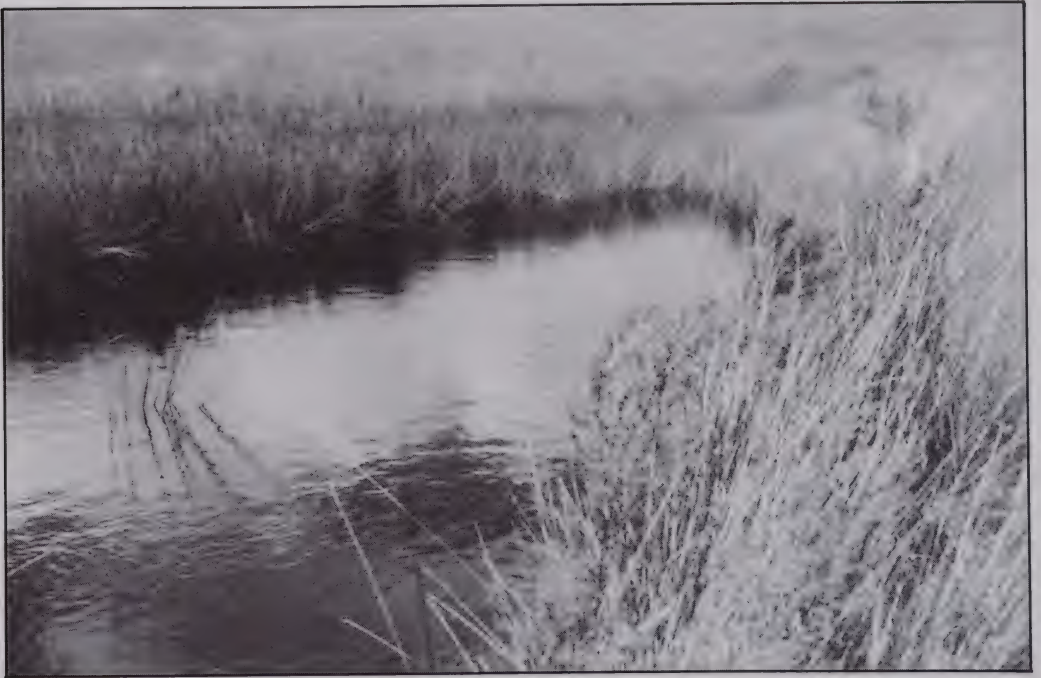
Fig. 5. Hukatere dam, southern end.
